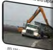
RD 150 provides emergency flood repair
