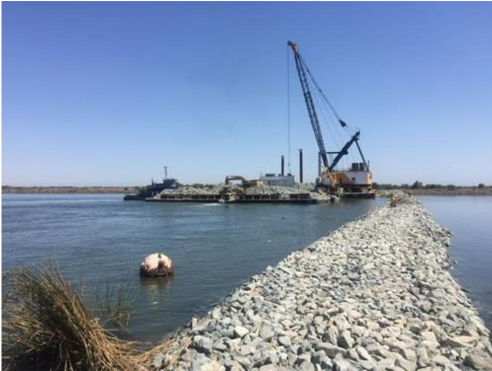
The Emergency Drought Barrier shown during construction in the Sacramento-San Joaquin Delta at West False River. The temporary 800-foot wide barrier is to control water salinity into the Delta and preserve water in upstream reservoirs.
